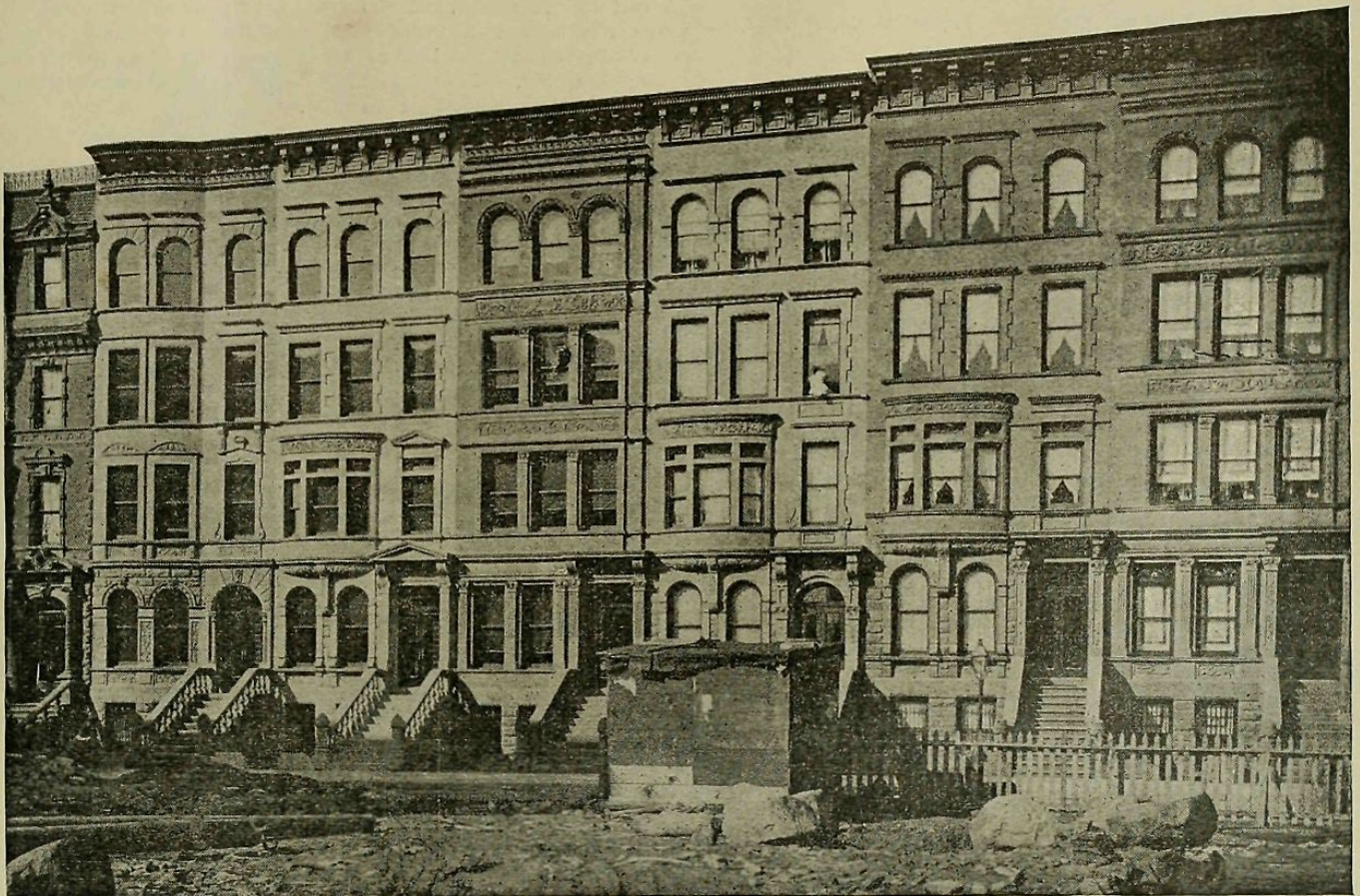
North Side of 92d Street, West of Madison Avenue.
