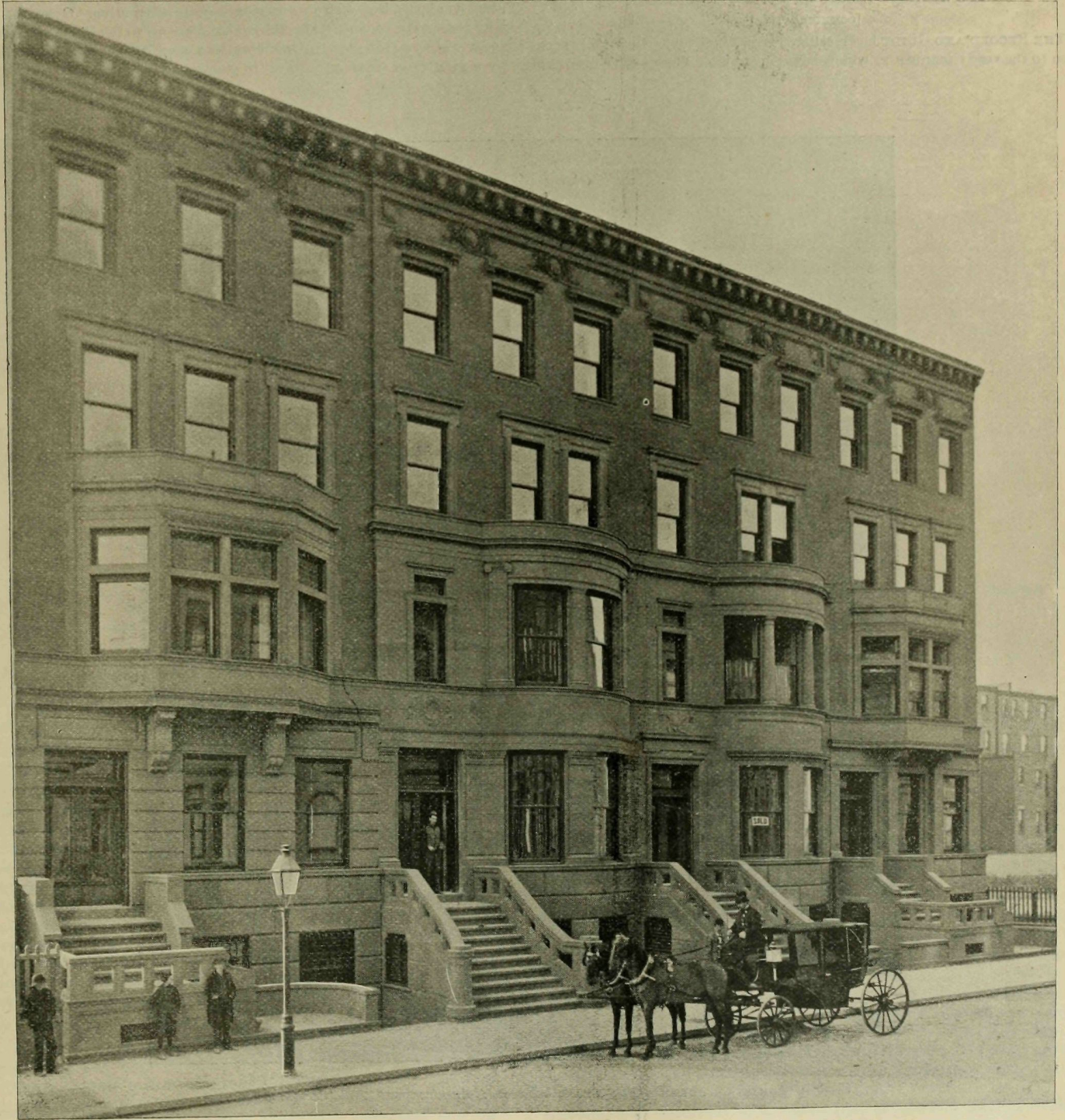
Residences on Seventy-fourth Street, near Central Park West.
