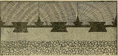
Composed of wood blocks, cemented and keyed to concrete foundation, forming a solid and immovable structure, through which no dampness or foul air can penetrate and no disease germs or filth can be secreted.
