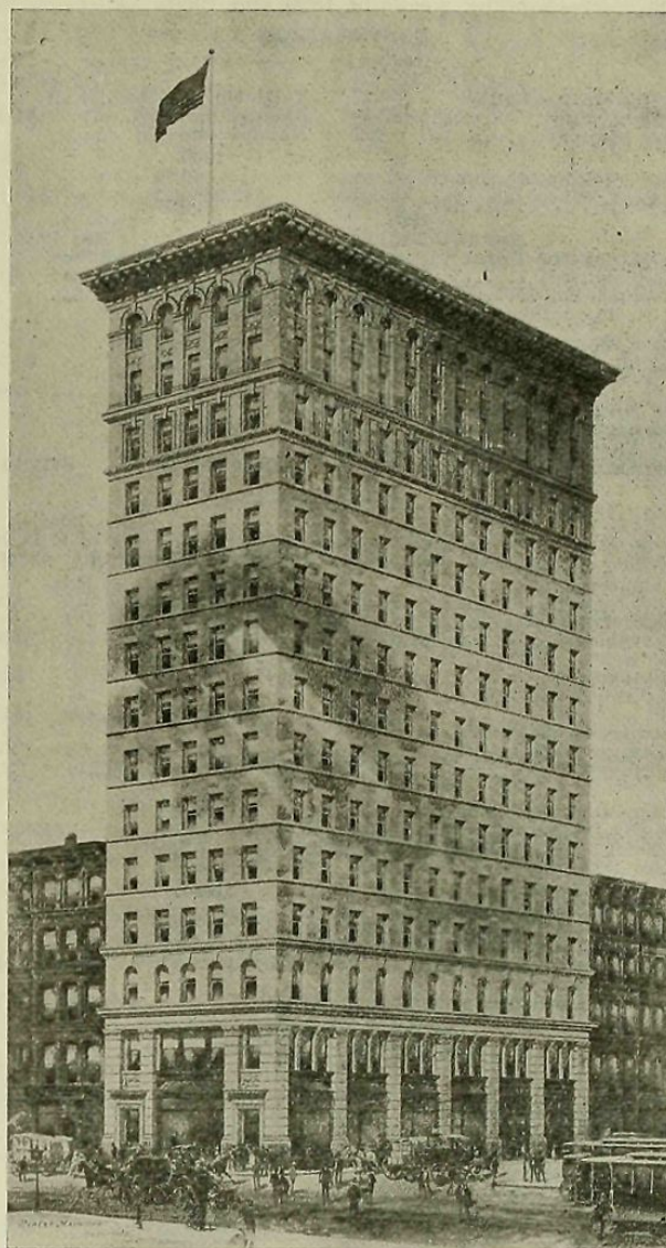
S. W. CORNER WALKER ST. AND BROADWAY. Robert Maynicke, Architect.
