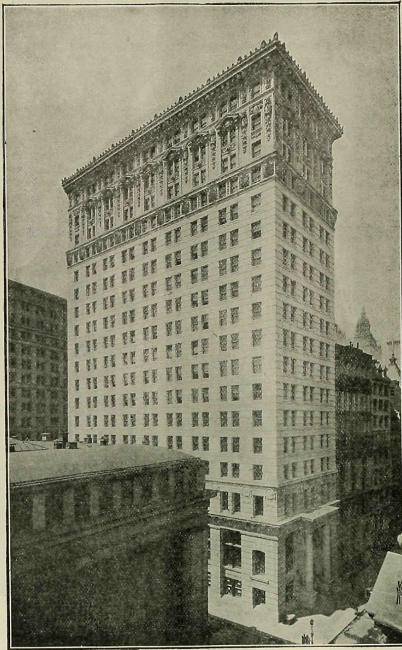
ATLANTIC MUTUAL BUILDING.
