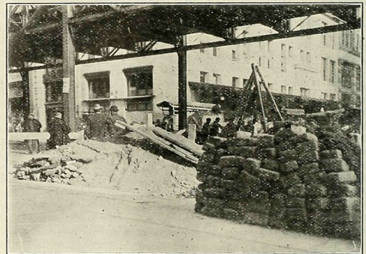
A SIXTH AVENUE OBSTRUCTION.
