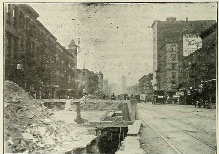
DIGGINGS IN 7TH AVENUE.
