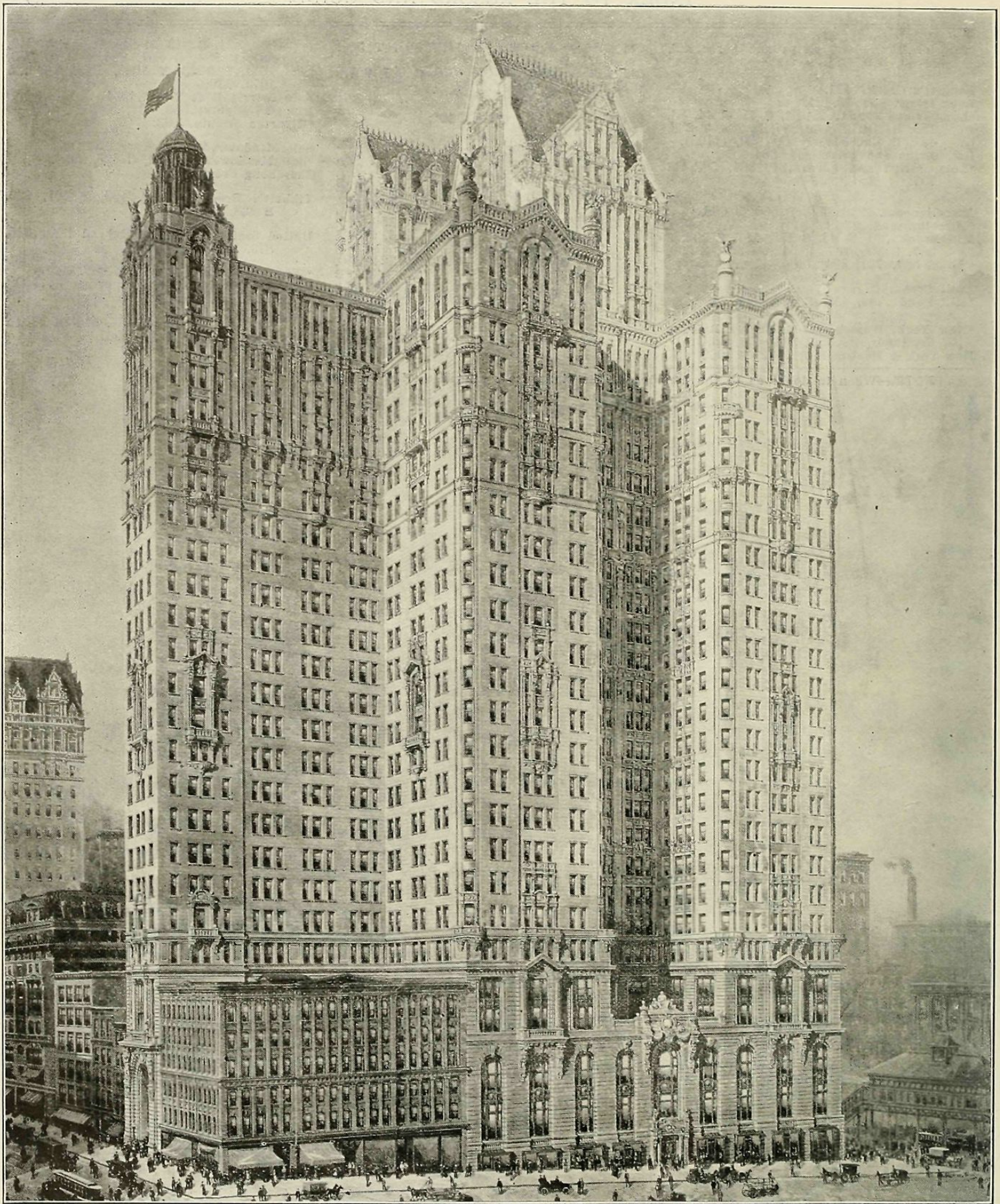
CITY INVESTING BUILDING (in course of construction), Broadway, Cortlandt and Church streets. Ready for occupancy May 1, 1908.
