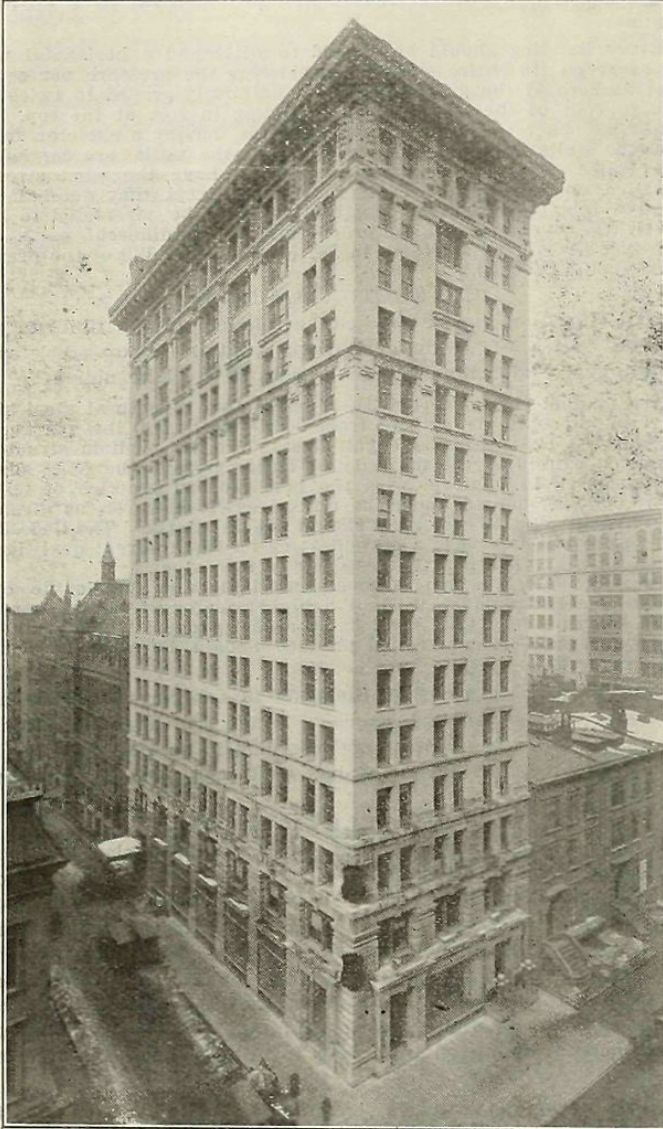
A MANHATTAN IMPROVEMENT—"STUYVESANT" BUILDING. Northwest corner 5th Avenue and 15th Street.
