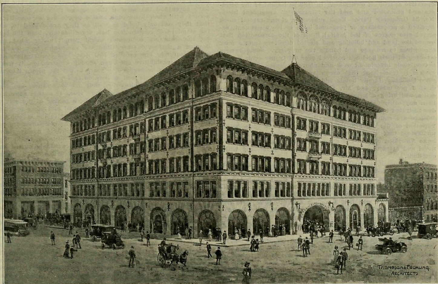
DESIGN OF THE BELMONT TUNNEL TERMINAL BUILDING AT LONG ISLAND CITY. Thompson & Frohling, Architects.
