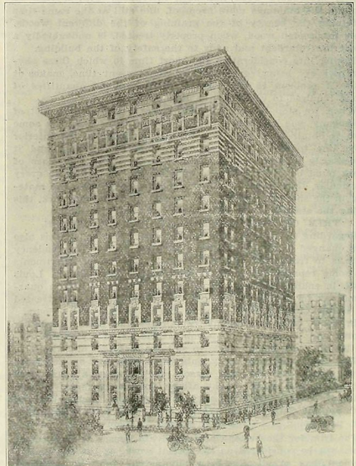
THE CLARENDON APARTMENT HOUSE. Riverside Drive and 86th st. Chas. E. Birge, Architect.
