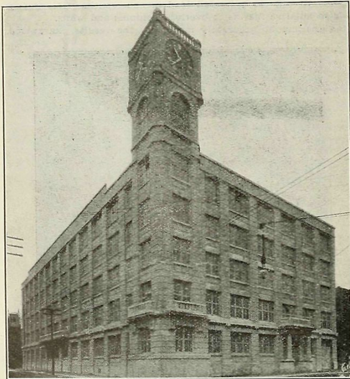
CONCRETE-STEEL MANUFACTURING BUILDING ERECTED FOR KEUFFEL & ESSER CO., IN HOBOKEN, N. J.
