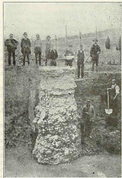
A COMPLETED PILLAR.
