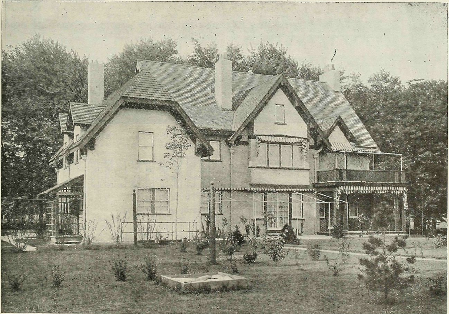
Ewing & Chappell, Architects.
