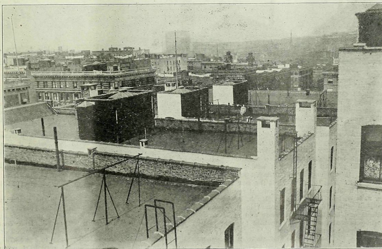
FIG. 6. NEW-LAW TENEMENTS, UPPER WEST SIDE, SHOWING NEARER VIEW OF COURTS, ROOF LINE AND GOOSENECK FIRE-ESCAPE LADDER TO ROOF.
