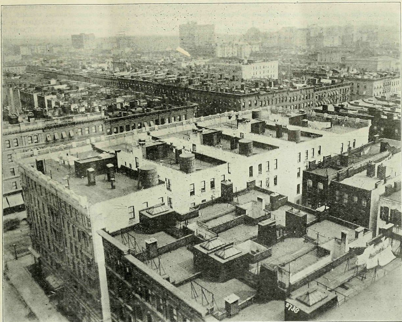
FIG. 5. BIRD'S-EYE VIEW OF FIVE NEW-LAW TENEMENTS, SHOWING LARGE OUTER COURTS CONNECTING WITH THE YARDS.
