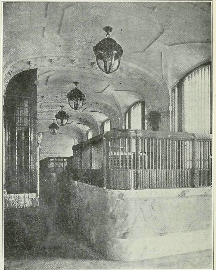
VIEW IN FIRST FLOOR BANKING ROOM. Importers and Traders National Bank.
