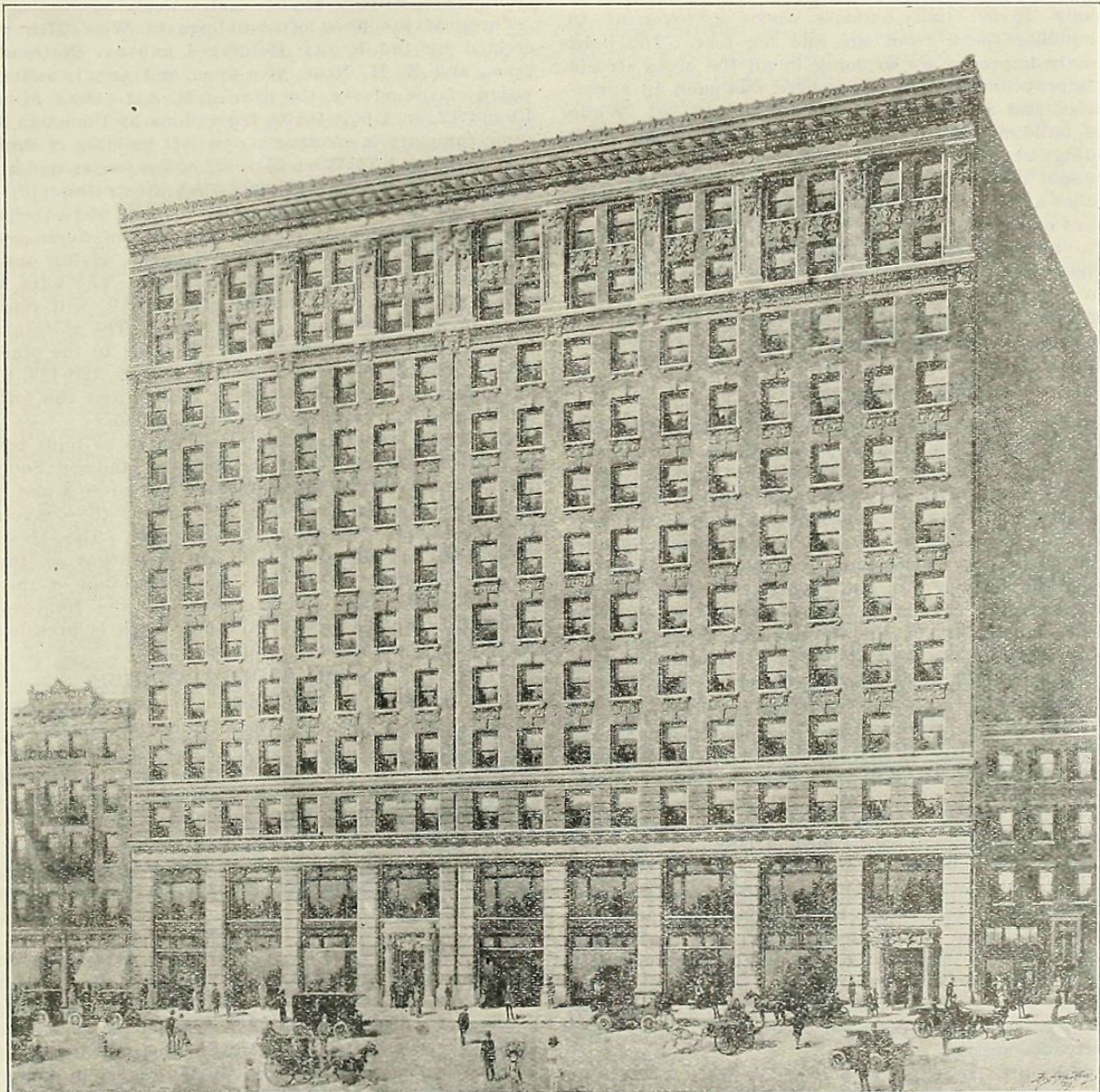
A WEST 27TH STREET IMPROVEMENT.
