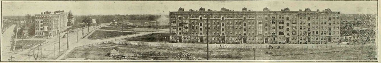
Looking north and west across portion of "A-Re-Co" district, showing building operations completed last year, with the Watson estate, where development work is beginning this year, in the background.
