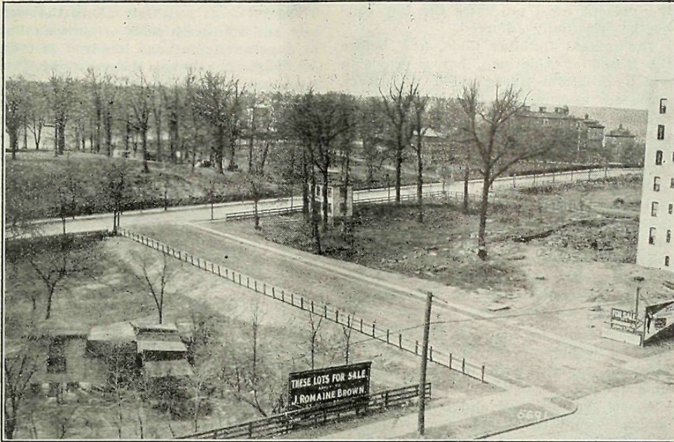
AN UNDEVELOPED NEIGHBORHOOD,—BUILDING OPERATIONS BEGINNING
