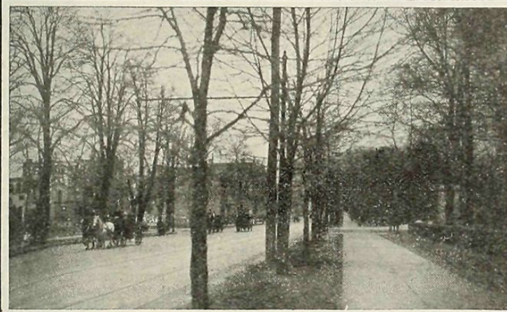
PROSPECT PARK WEST AT THIRD STREET.
