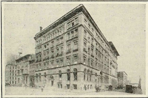
Exterior Brick Walls Finished with Summit Cement Paint. Post Graduate Hospital
