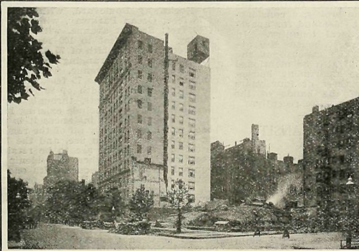
WEST END AVENUE, LOOKING NORTH FROM 83D STREET. The corner now vacant is being excavated for a twelve-story apartment house.
