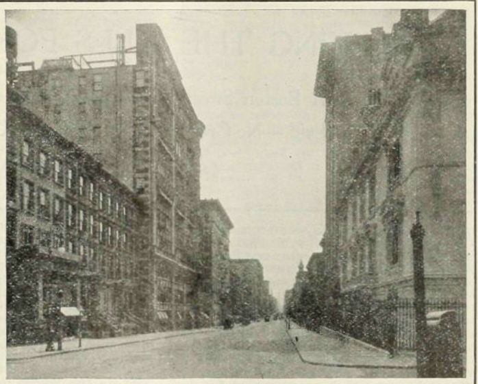
MADISON AVENUE, LOOKING SOUTH FROM 67TH STREET. Transitory conditions are apparent here. On the left is the only store within three blocks, and some modern apartments among old brownstone dwellings.
