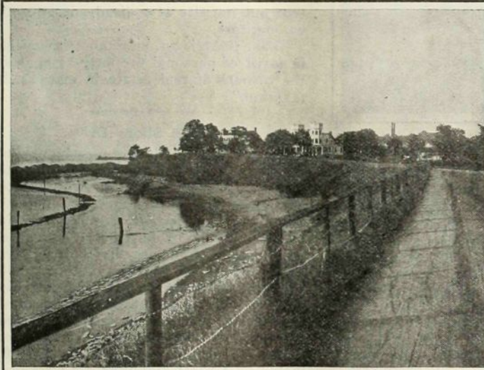
WORK ON SHORE ROAD IMPROVEMENT AT 77TH STREET.
