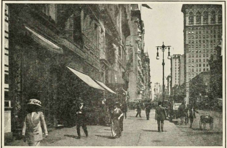
A FIFTH AVENUE SIDEWALK CLEAR OF ENCROACHMENTS.
