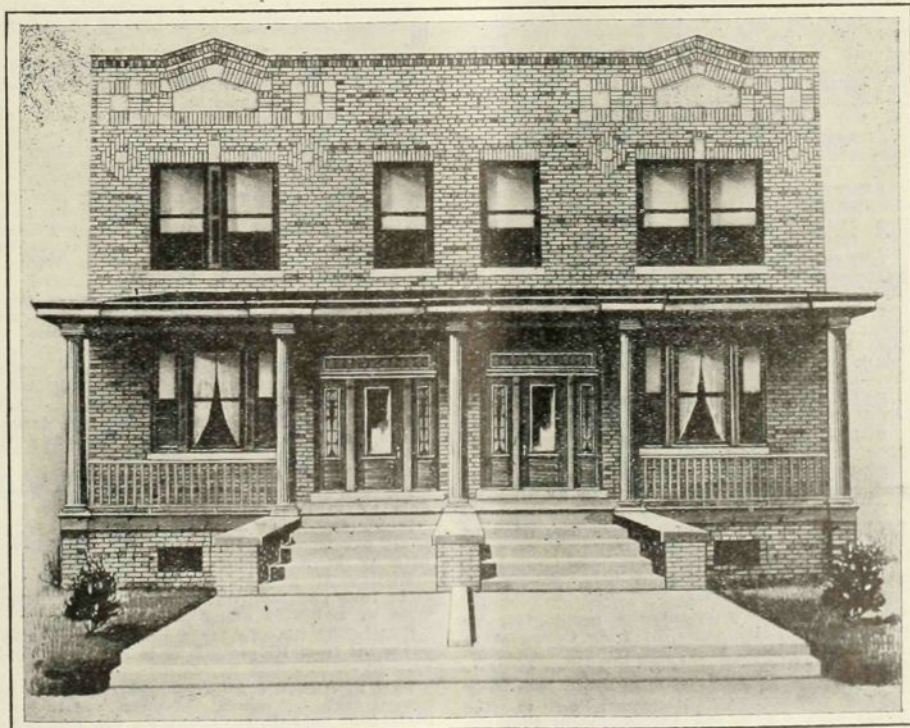
A PAIR OF "ALCO" HOUSES, TYPICAL OF FIFTY NOW NEARING COMPLETION ON 67TH STREET, BROOKLYN. THE METROPOLITAN LIFE INSURANCE CO. INSURES BOTH MORTGAGES IN CASE OF THE PURCHASERS DEATH.
