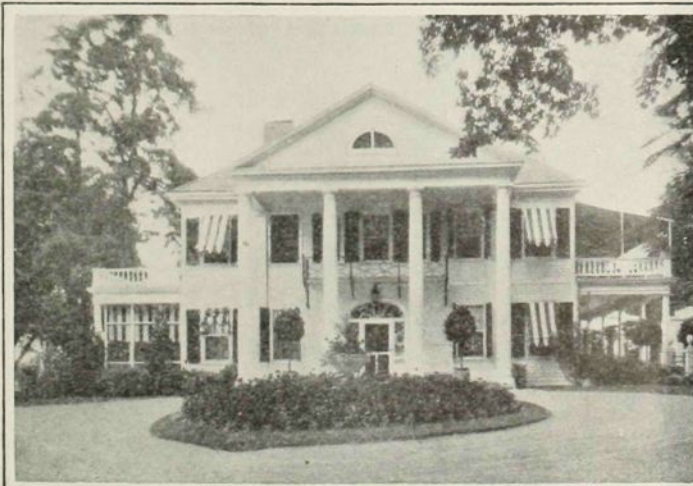
A COLONIAL RESIDENCE AT KENSINGTON.
