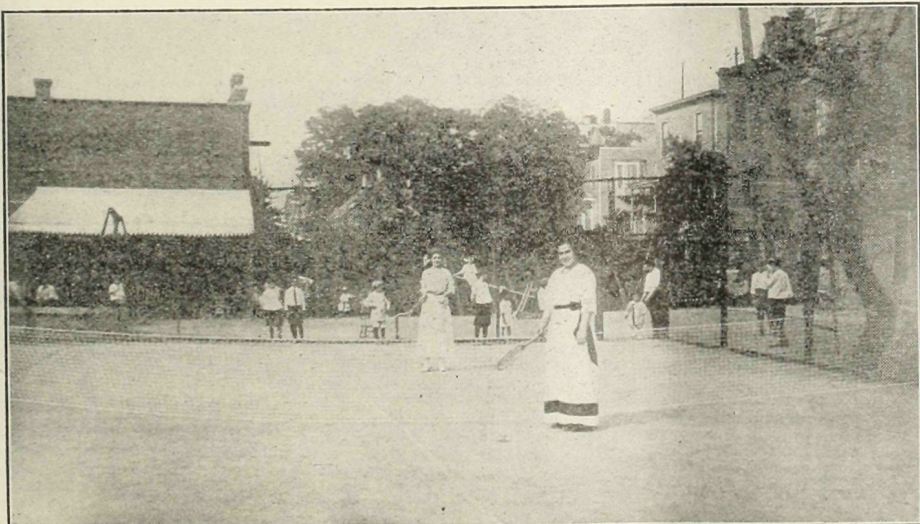
TENNIS COURTS ON FRANKLIN AVENUE, BRONX.
