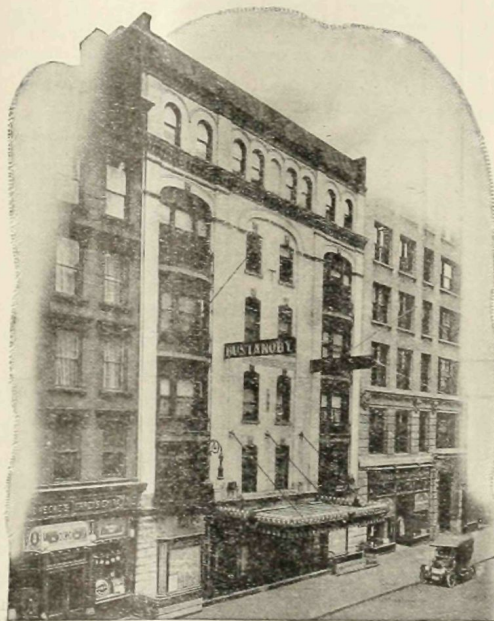
Bustanoby's Restaurant, 110 W. 39th St., New York City. A Kewanee Water Heating Garbage Burner is used to burn garbage and refuse and provide the hot water supply.
