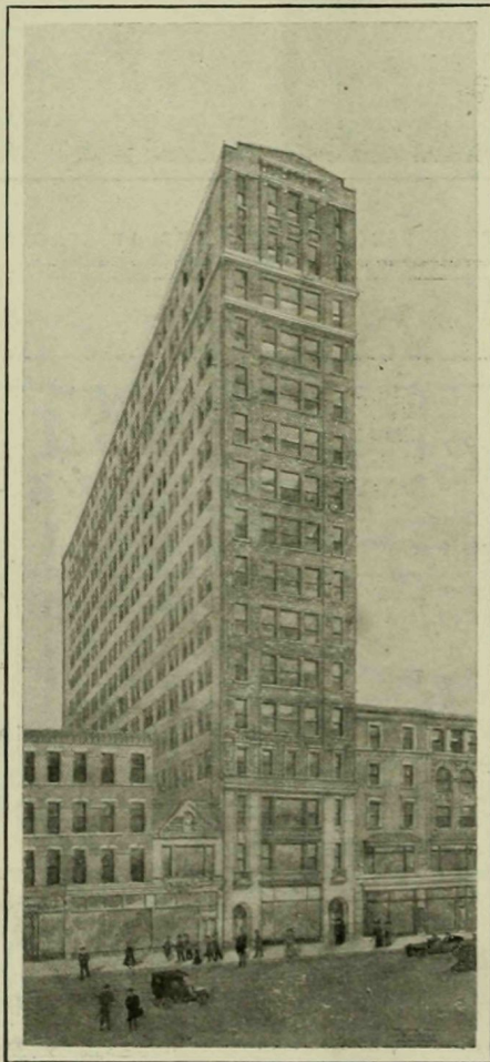
1237 AND 1239 BROADWAY. S. Walter Katz & I. G. Feiner, Arch'ts. Owner and Builder, Isaac A. Hopper, Inc.,
