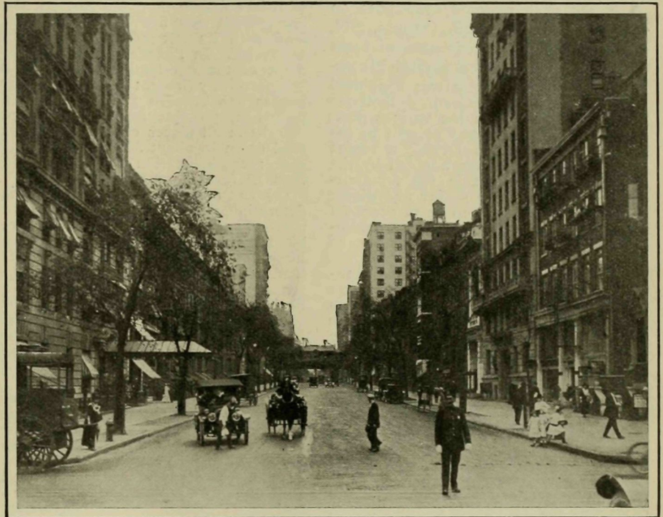
VIEW OF 72D STREET, EAST FROM BROADWAY.
