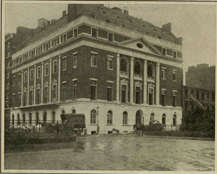
Norcross Bros., Builders.
