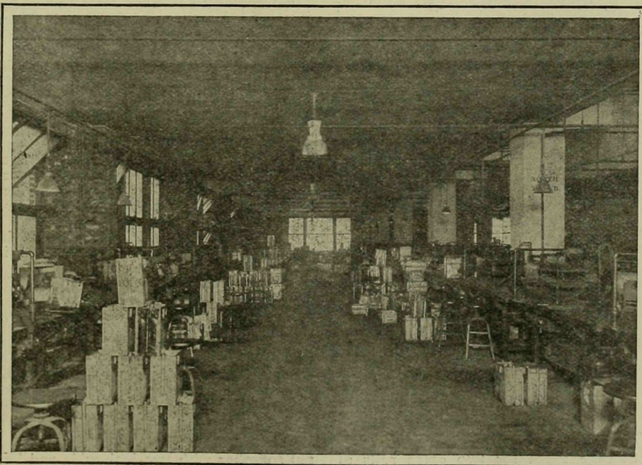
FACTORY LIT BY GAS.
