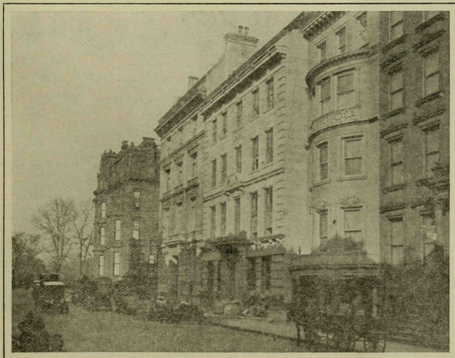
Residence now under construction at 7-9 East 61st Street for John T. Pratt. Charles A. Platt, is the architect and James McWalters & Son the general contractors.
