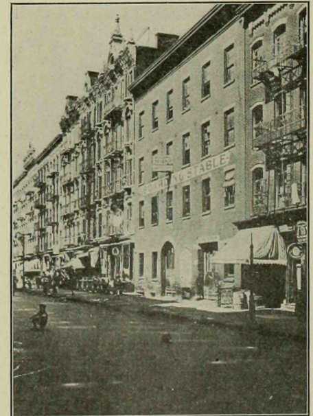
NO. 6.—THIS BLOCK IN 11TH STREET IS DEFILED AS A HOME FOR MEN BY THIS STABLE FOR HORSES.
