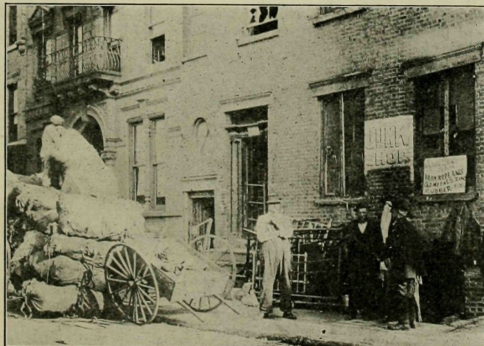
FEW WOULD SELECT THIS TENEMENT IN MORTON STREET AS A HOME, IF HE GLIMPSED THESE JUNKMEN.
