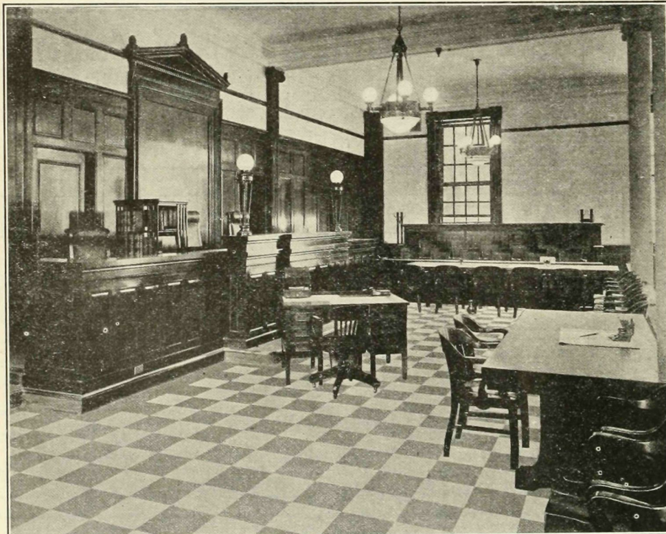
MIDDLESEX COUNTY COURT HOUSE, NEW BRUNSWICK, N. J., W. H. BOYLAN, Architect
