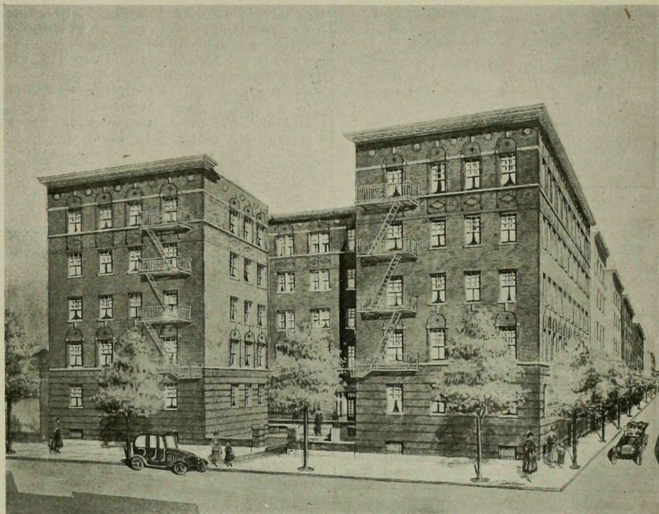
Niewenhou Bros., Builders. MODERN APARTMENTS UNDER CONSTRUCTION IN THE BRONX.
