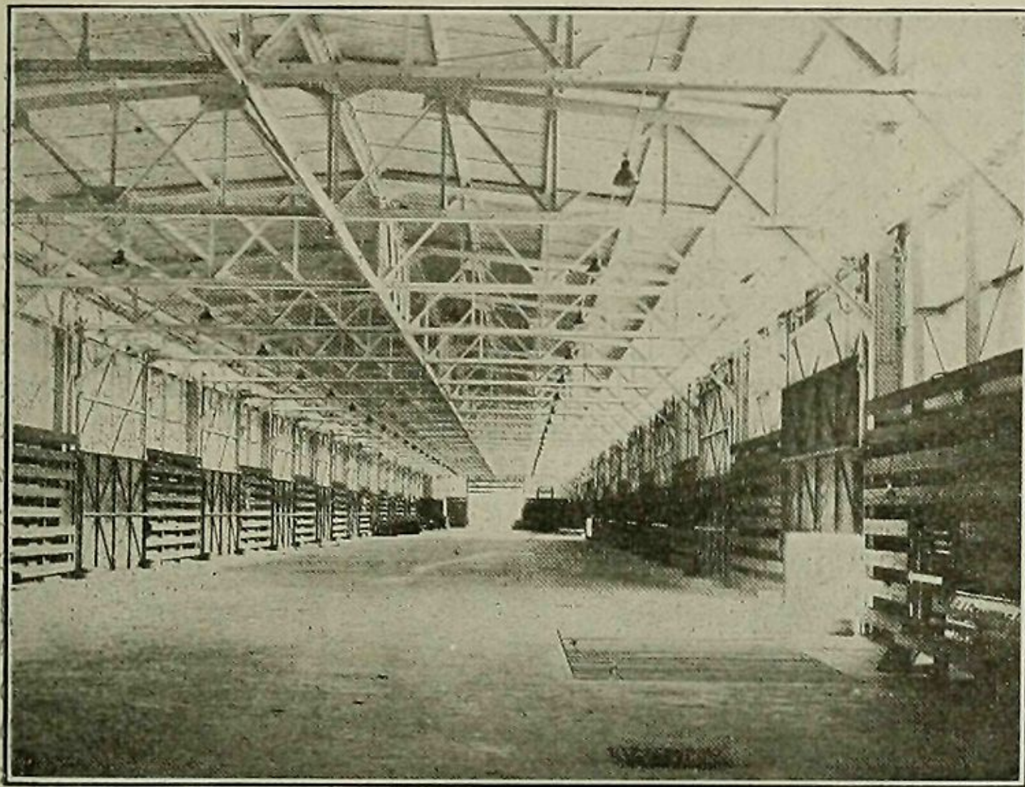
INTERIOR VIEW OF PIER SHED.
