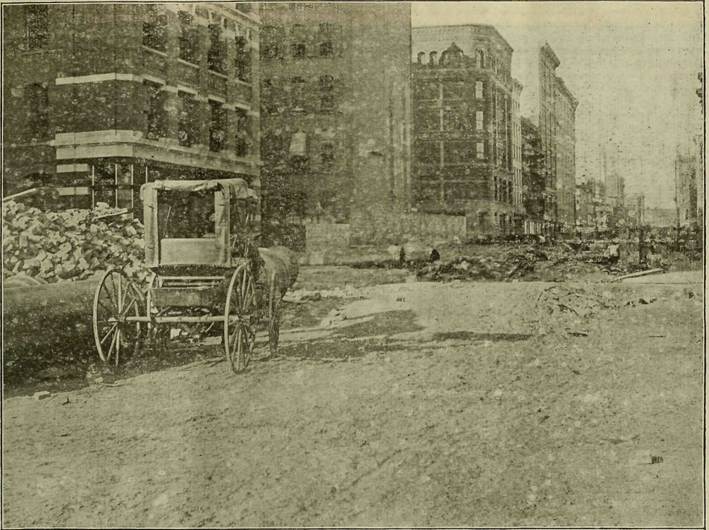
ELM STREET "IMPROVEMENT," LOOKING NORTH, FROM JERSEY STREET.
