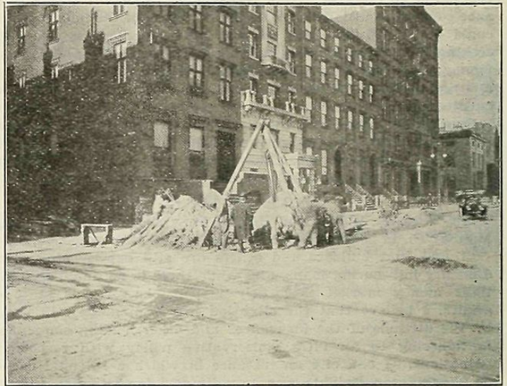
1—OBSTRUCTIONS AT FIFTH AV AND EIGHTH ST.
