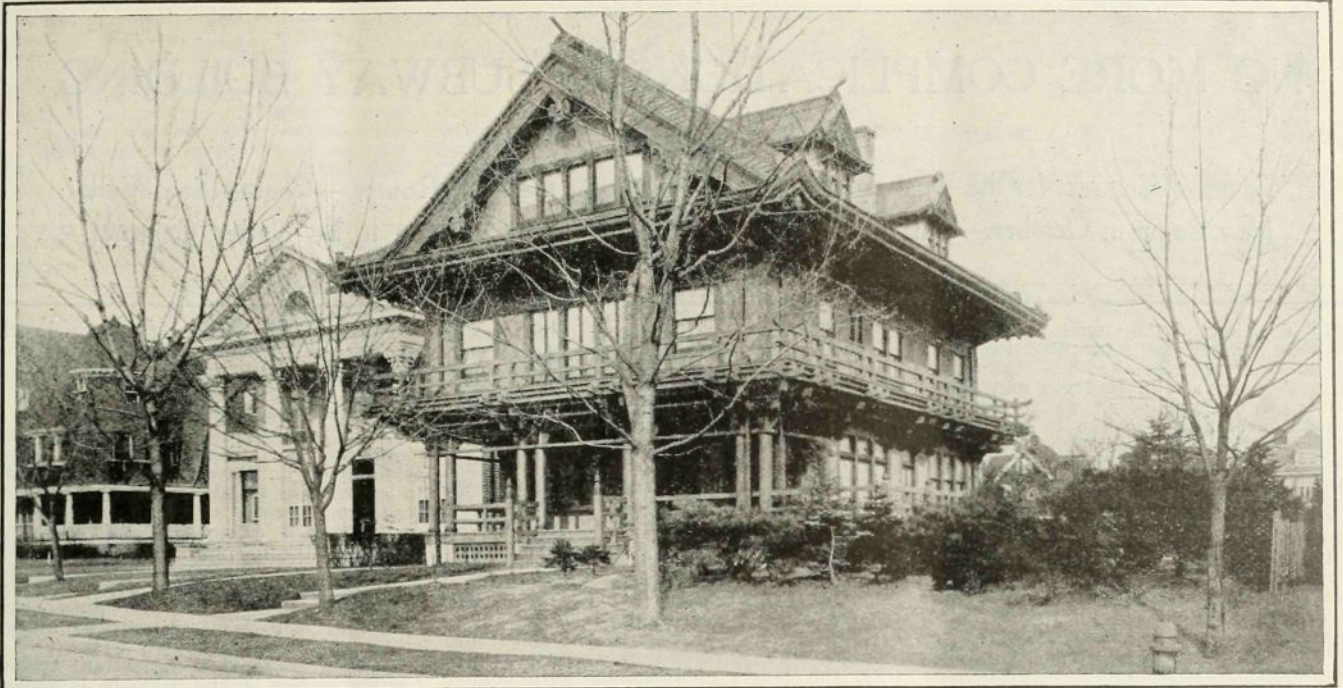
EXAMPLE OF JAPANESE ARCHITECTURE.—This building, though attractive, remained unsold for a number of years after its erection. It is too conspicuous, too much of a departure from accepted types, and was finally sold at far less than its cost of production. Prospect Park South, Brooklyn, N. Y.
