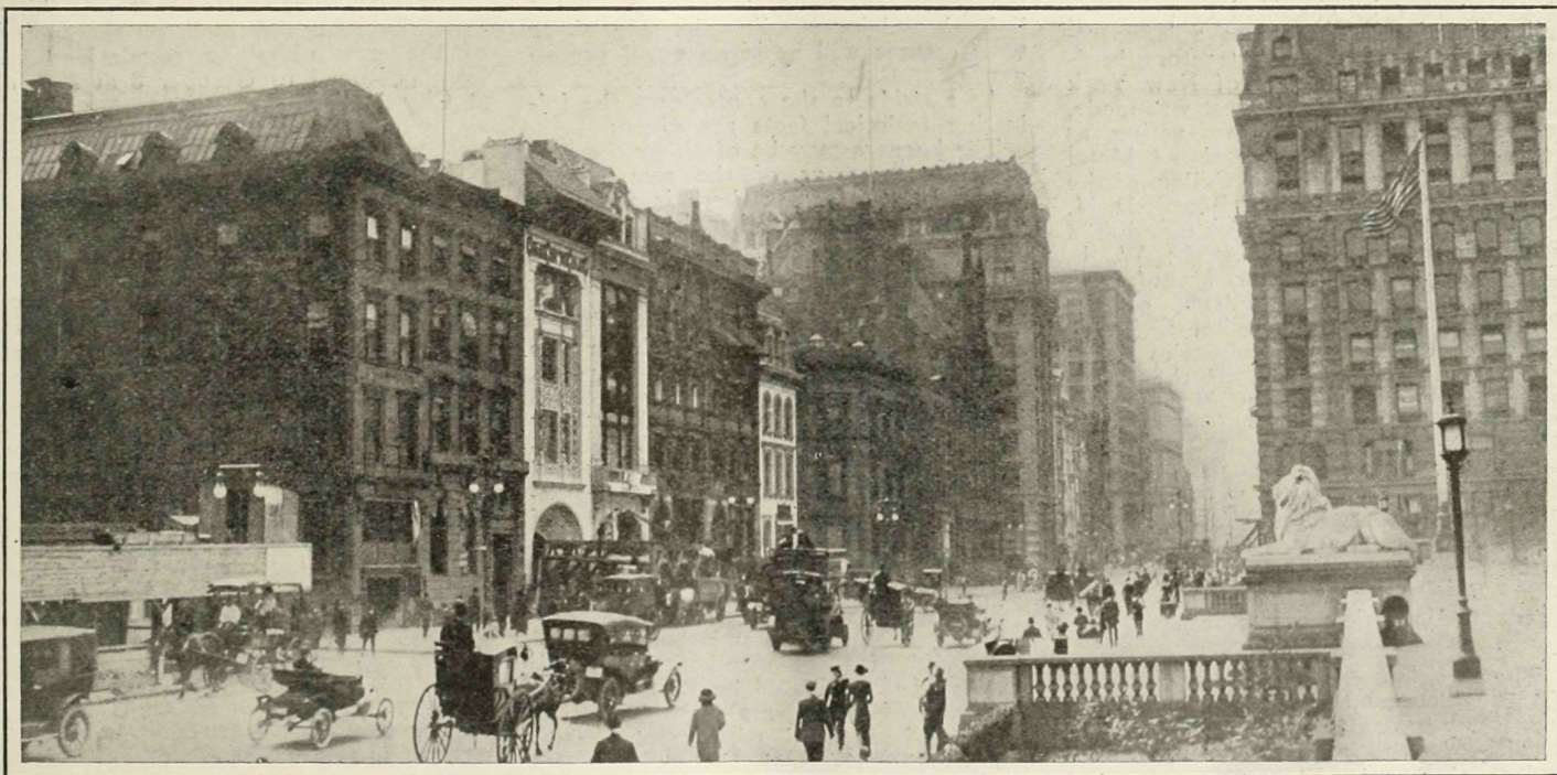
FIFTH AVENUE, SHOWING SITE OF PROJECTED BUILDING.
